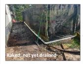
Before the blue metal (all 4 tonnes of it) was laid, it was necessary to remove large quantities of mud that sat on the rock slabs. Once that was done, the blue metal stopped sinking into the quagmire and the path began to take shape!
